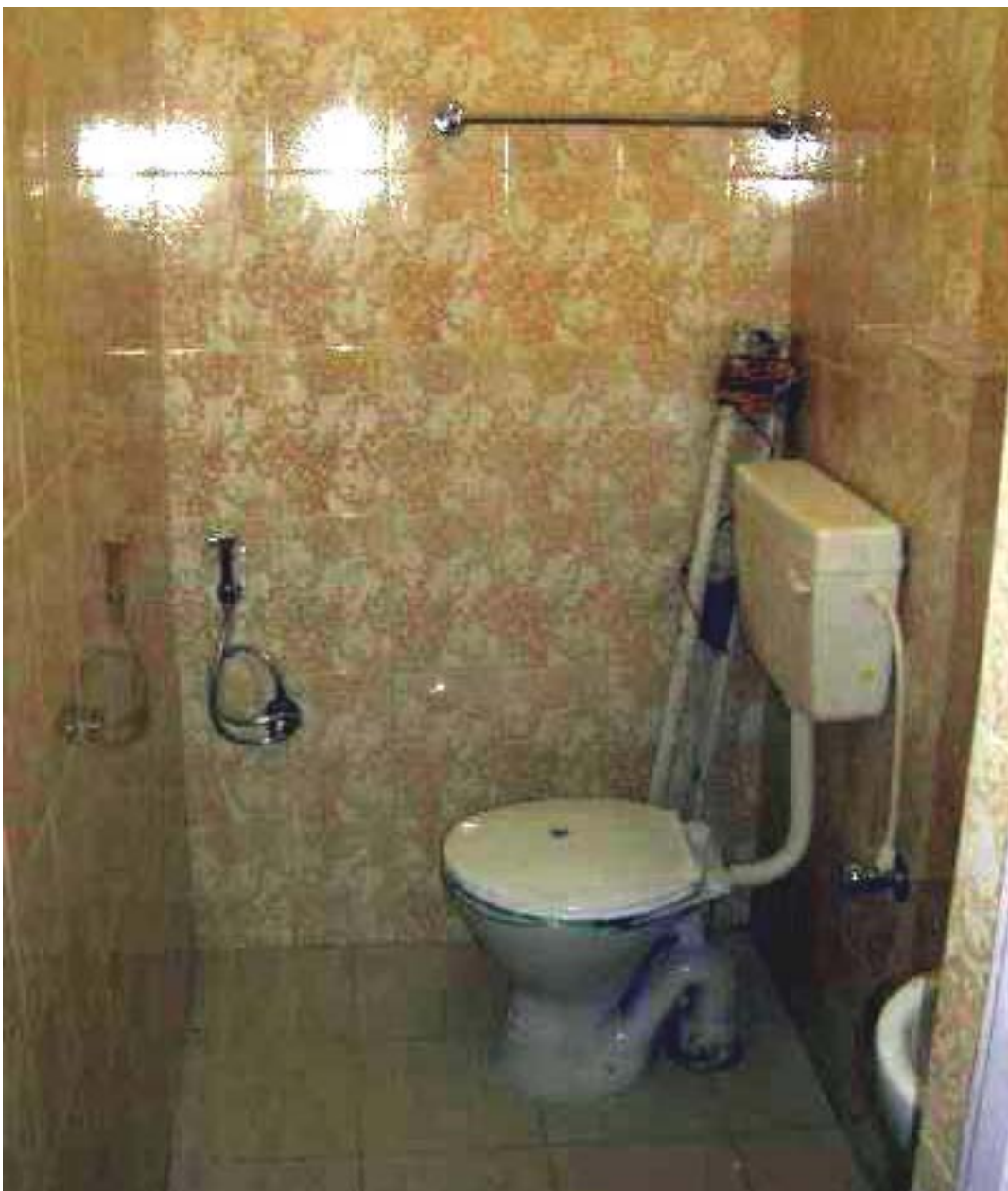
The new shower room
